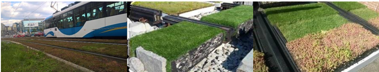
Image 4: Pilot grass planting in tramline strips
